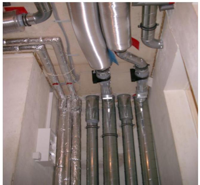
**Figure 5: Building services piping under the ceiling of the corridor in the flats**
